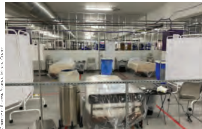
The Renown COVID-19 field hospital photographed under construction in Reno.
