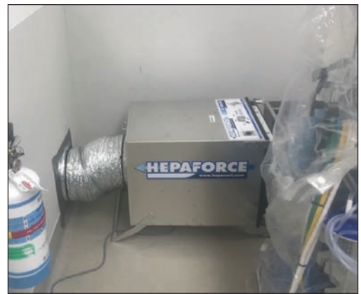
FIGURE 3 Portable Filtration System With Filtered Exhaust Directed Into Ventilation Return Columns
