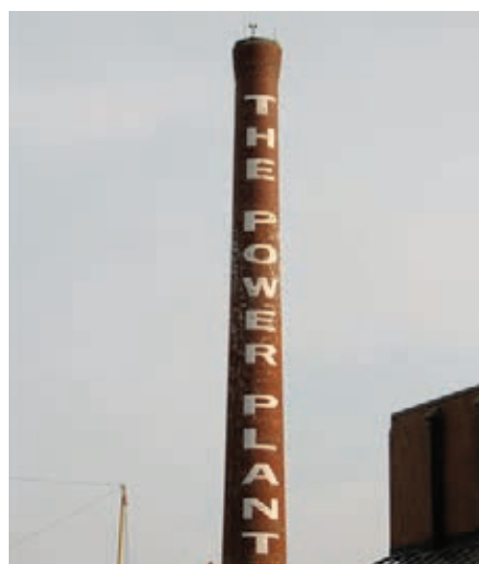
The Power Plant
